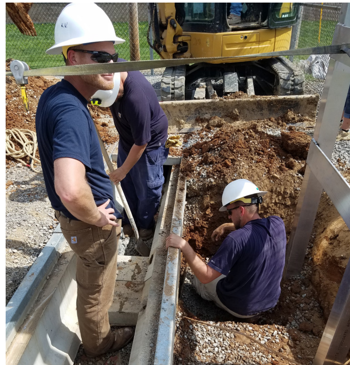
INSTALLING CONDUIT AT OUR “BARTON” SUBSTATION
