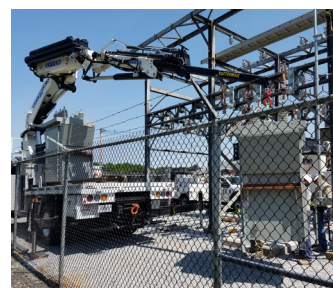
INSTALLING NEW BREAKERS AT “BARTON” SUBSTATION
